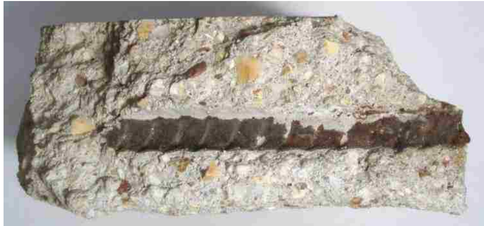
Figure 3.19: Red rust observed along the inner surface of a segment of 50/50 enamel that remained attached to a section of concrete.
