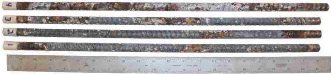
Figure 3.18: A typical set of uncoated reinforcing bars after being removed from a ponding specimen.
